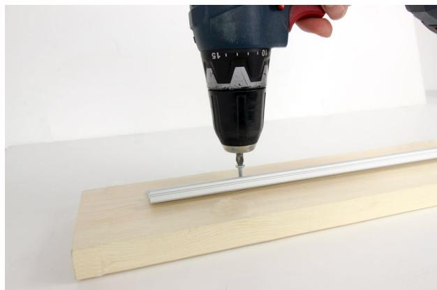
2. Screw in the wire mounting clip. For the best support, install the clip within one inch of the end of the track.
