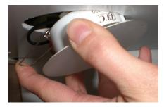
4. Installing the screw mount version: Remove cover by twisting counter clockwise. Mark location of screw holes and pre-drill. Screw in fixture and re-install cover by twisting clockwise.
